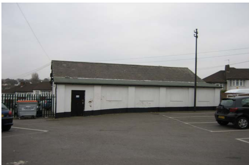
Rear view from Church Farm
