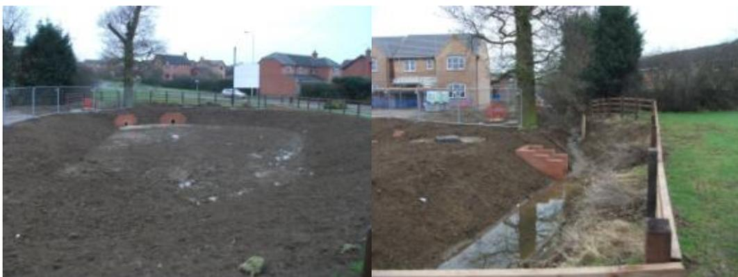
**Figure E2-9 Example of an offline storage structure under construction**
