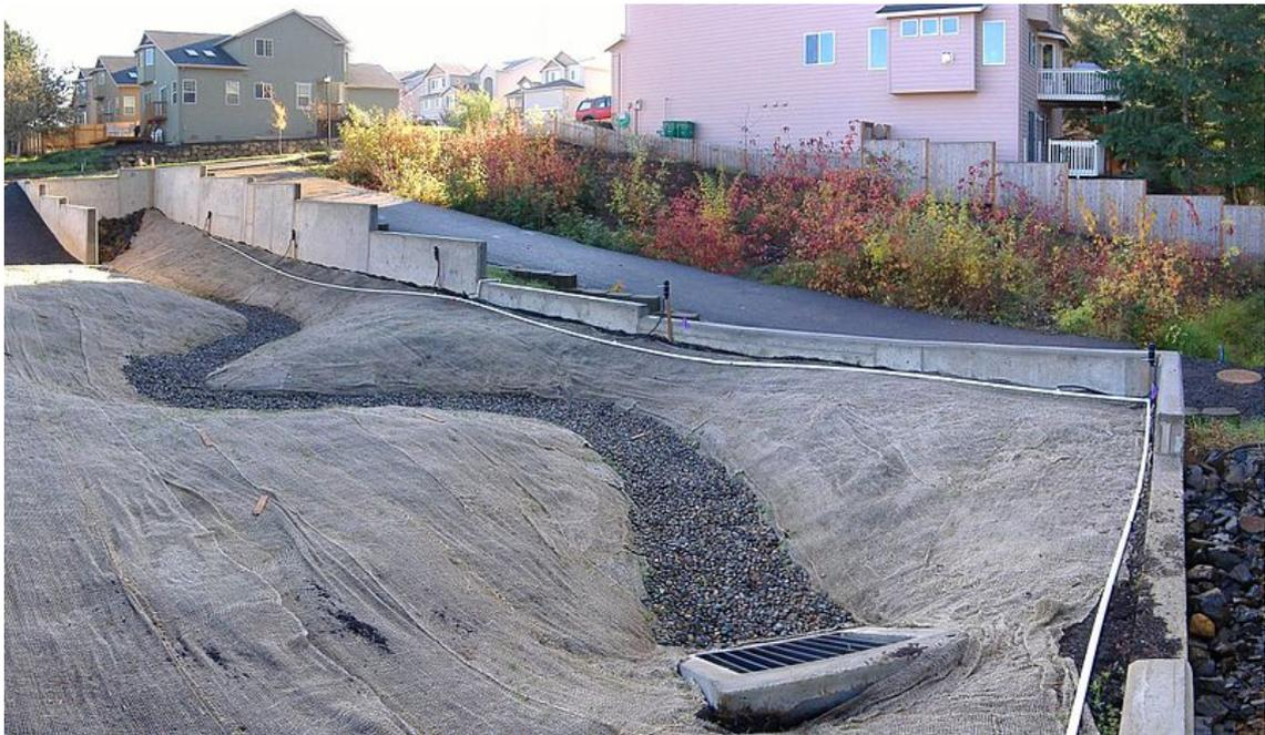
**Figure E2-7 Example of swale under construction (completed swale shown in background)**
