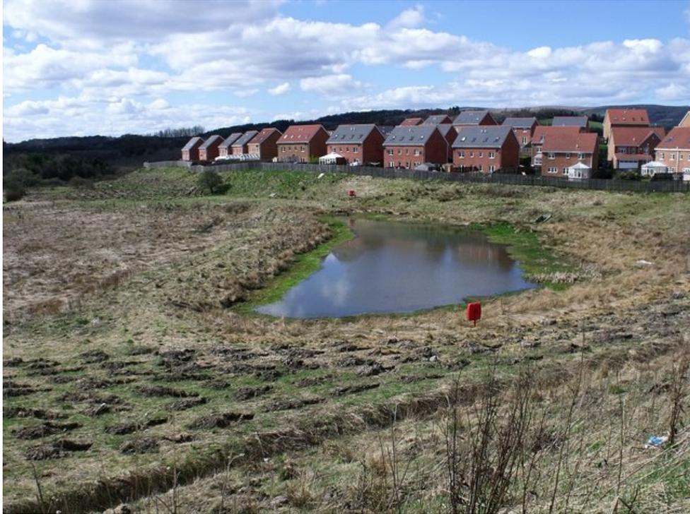
**Figure E2-8 Example of Detention Basin © Copyright BJ Smur<sup>vi</sup>**
