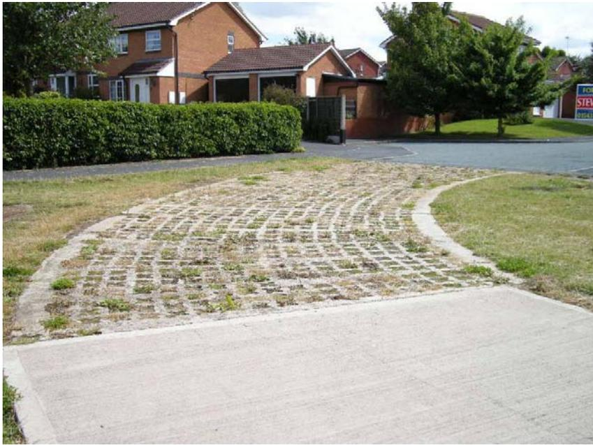
**Figure E2-5 Example of permeable paving**
