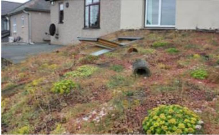
Figure E2-1 Example of a residential green roof (Ecotips, 2010<sup>1</sup>)
