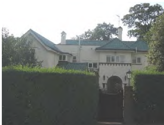
Mote Lodge, Nan Clarks Lane
