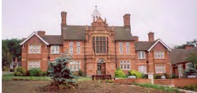
The Grade II listed Marshall Hall forms the centrepiece of the Retail Trust estate
