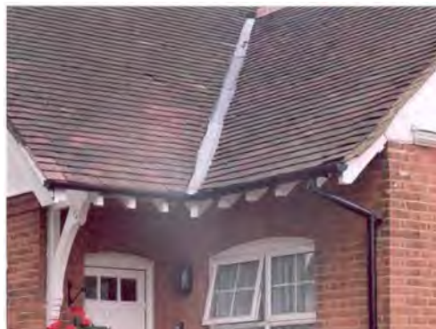
Over-sailing eaves with exposed rafter feet
